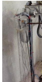
Gambar 3.4 Leg (Kaki Electric Container Crane). Sumber: Peneliti (2017)
