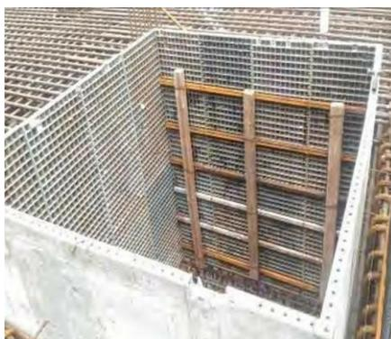
. Gambar 10 Bekisting ( fit lipt ) pondasi raft
