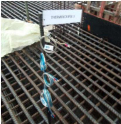
**Gambar 3.2 Thermocouple**
